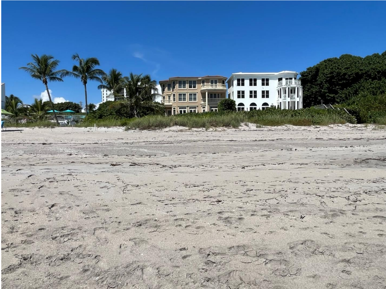
Photo 14. West view of the two single family homes and a portion of the Boca Highland Beach Club. Note the elevation of the dune relative to the adjacent Milani Park parcel.
