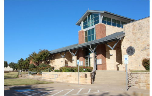
HICKORY CREEK TOWN HALL
