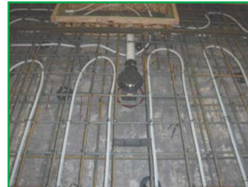
Hydronic Floor - Freeze Protection
