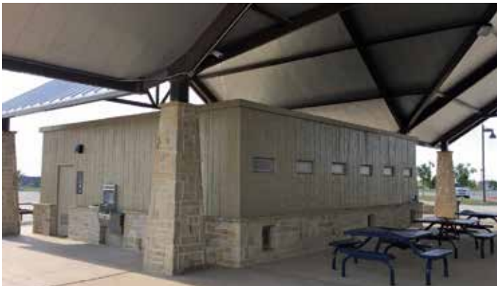
Flush restroom with custom stone texture and flat roof
