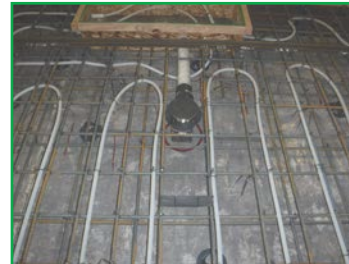
Hydronic Floor - Freeze Protection
