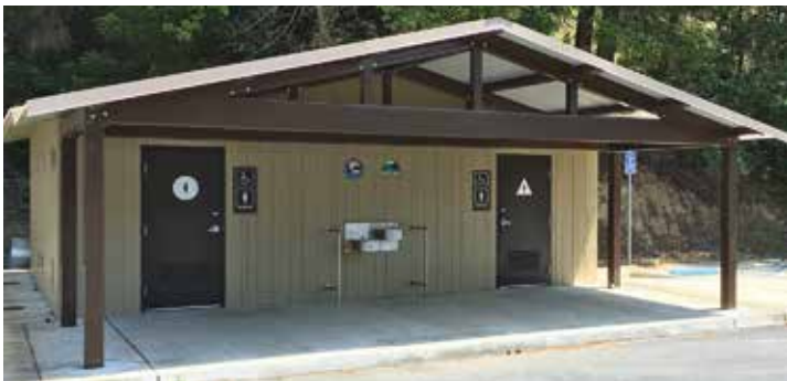
Flush restroom with custom awning
