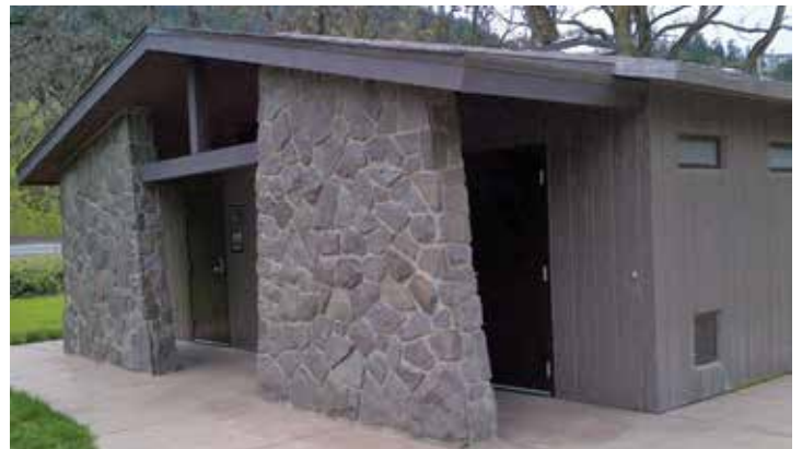
Flush restroom with custom covered entry
