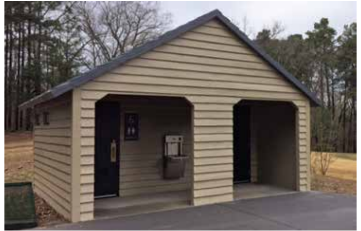
Flush restroom with custom golf cart shelter
