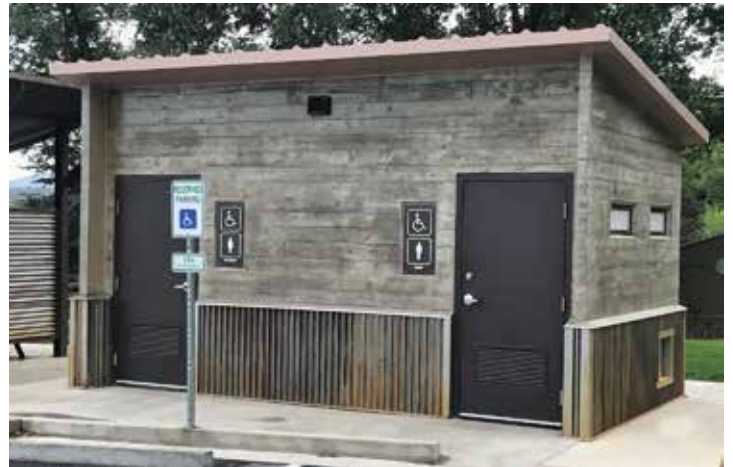
Flush restroom with custom texture and roof pitch
