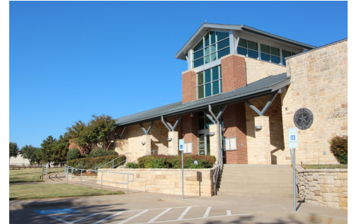
HICKORY CREEK TOWN HALL
