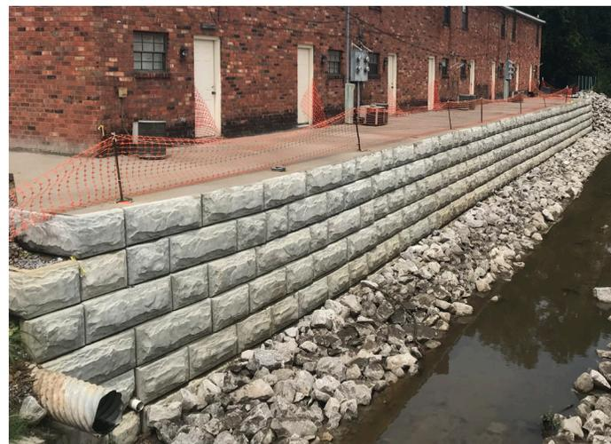
**The mass in each modular block helps resist deflection - allowing compactors and other heavy equipment to operate immediately behind the back of the units. By compacting to the back of the unit, Stone Strong Systems avoids the built-in defect small block systems have with backfill.**
