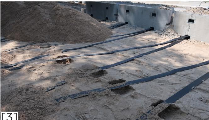
Paraweb straps can be driven over with equipment after covering with minimum 3 inches of backfill.
