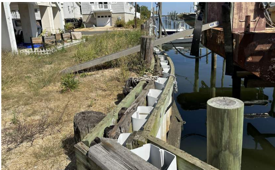
Photo 21: Section C , Westerly Bulkhead, View from grade
