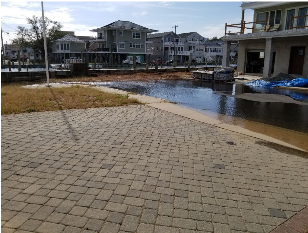
Flooding observed at Recreation Place (9-30-2019)(Provided by William Brunt)
