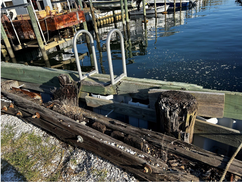
Photo of the Southerly Bulkhead (10-21-2024)(Provided by HGA)
