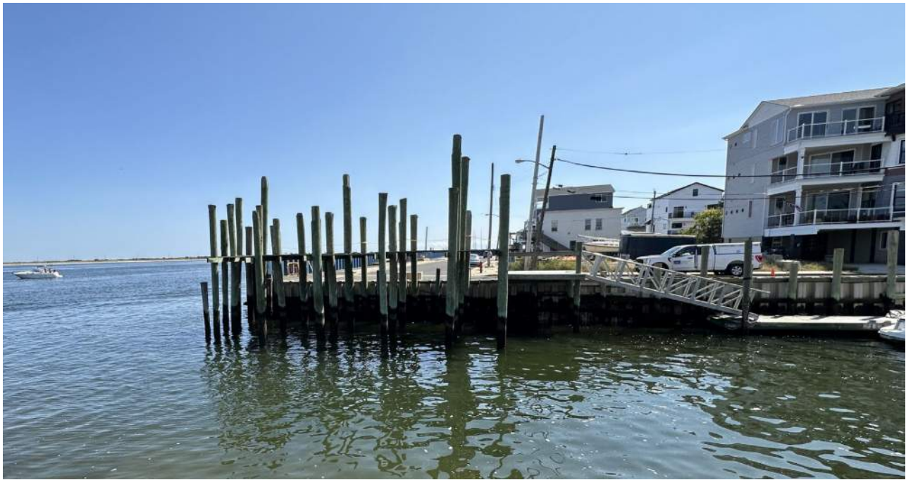
Photo 40: Section D , Easternly Dock, Viewed across Marina from Westerly Bulkhead
