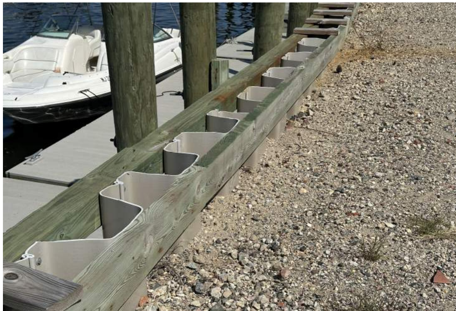
Photo 2: Section A , Easternly Bulkhead, Viewed from Grade
