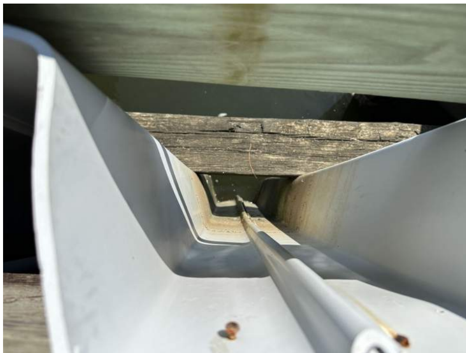
Photo 23: Section C , Westerly Bulkhead, Viewed down Sheet Pile, View 1
