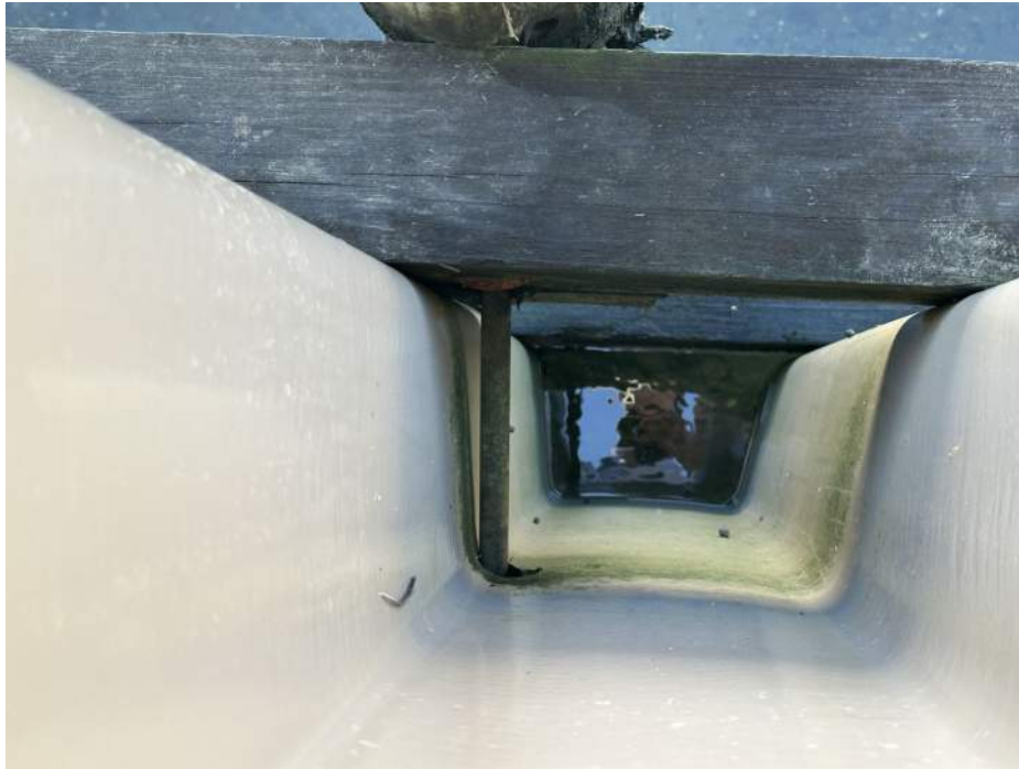
Photo 10: Section A , Easternly Bulkhead, Viewed down Sheet Pile
