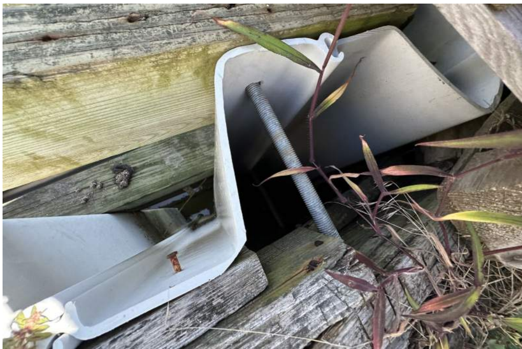
Photo 19: Section B , Southernly Bulkhead, Vinyl Bulkhead Connection
