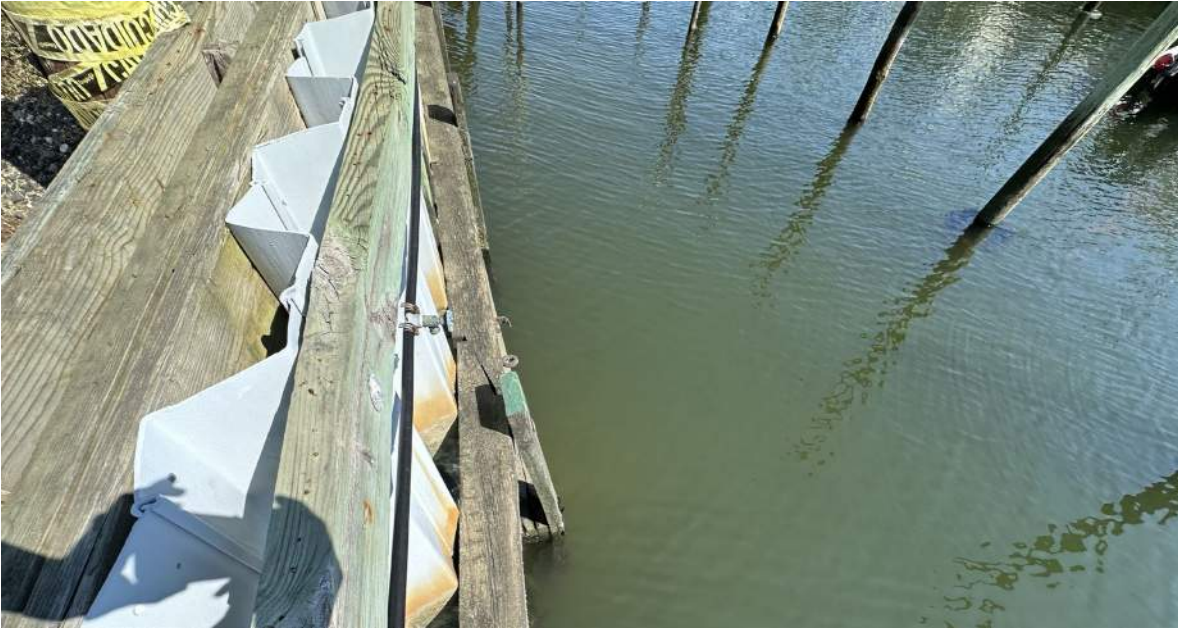
Photo 34: Section C , Westerly Bulkhead, Bowed Out Bulkhead Repair, View 1
