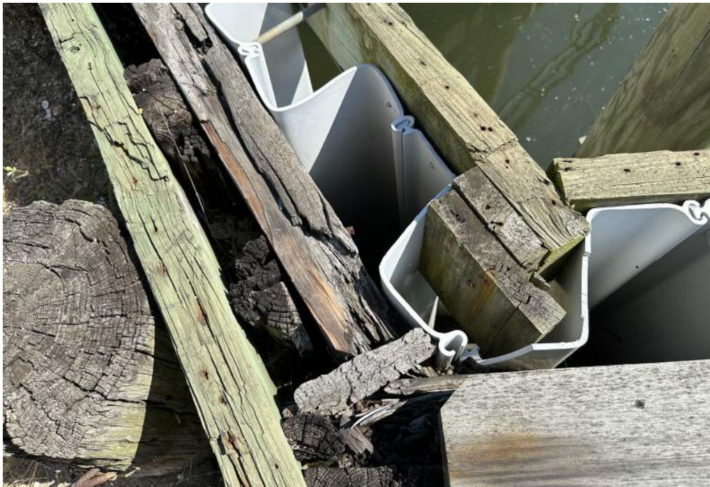
Photo 22: Section C , Westerly Bulkhead, Corner Connection to the Southernly Bulkhead
