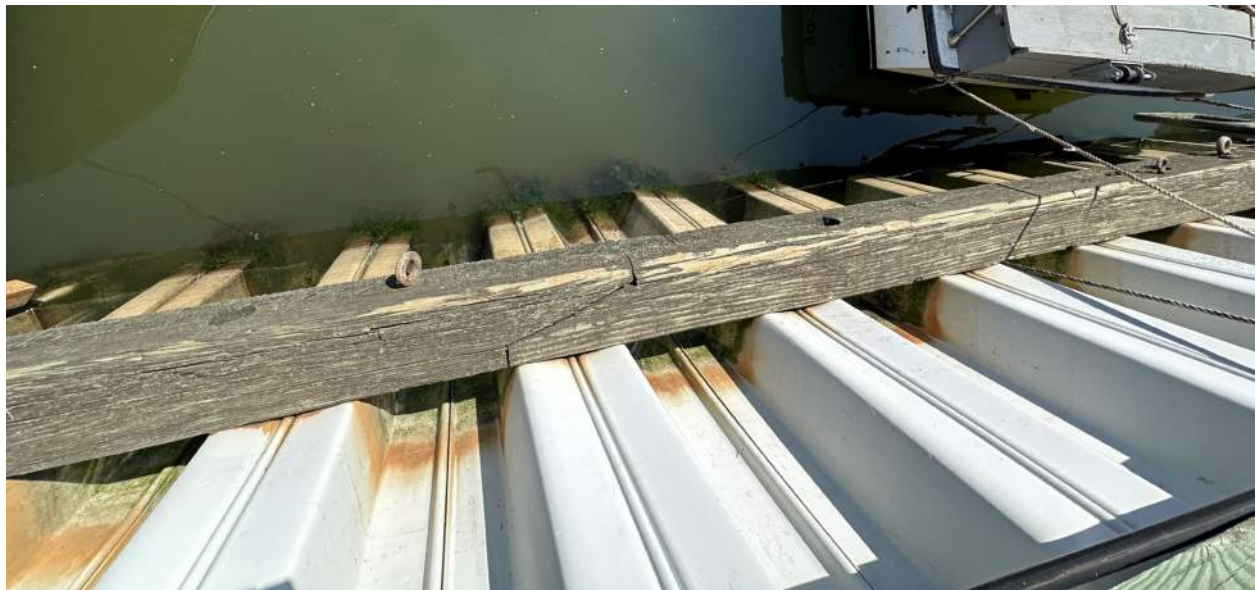
Photo 29: Section C , Westerly Bulkhead, Single Waler on Vinyl Sheet Pile, View 1
