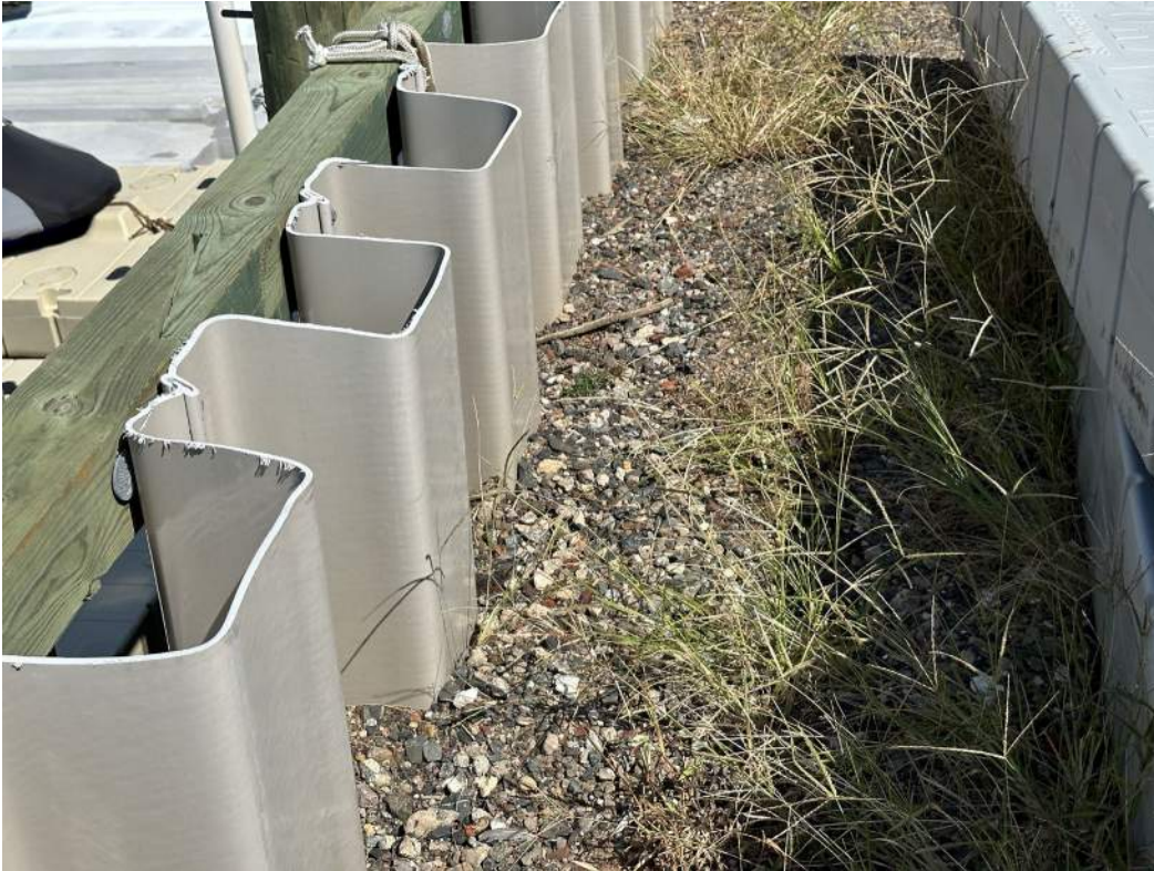
Photo 8: Section A, Easternly Bulkhead, View 2
