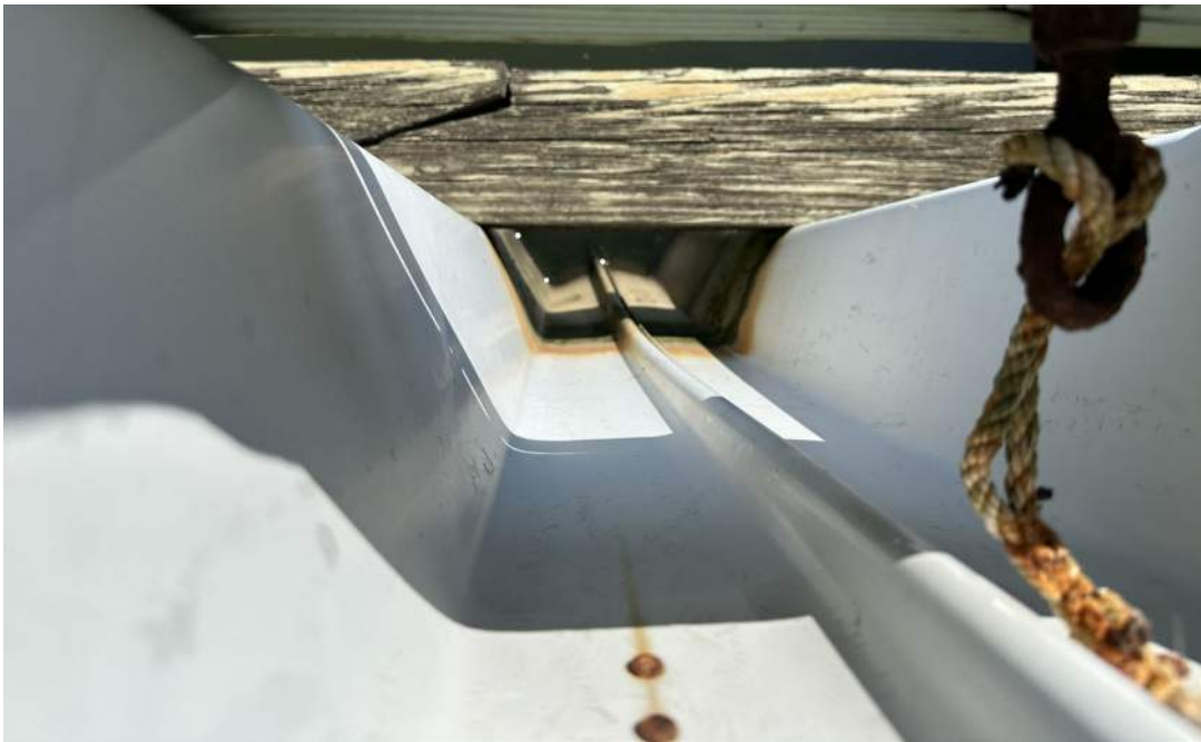
Photo 24: Section C , Westerly Bulkhead, Viewed down Sheet Pile, View 2
