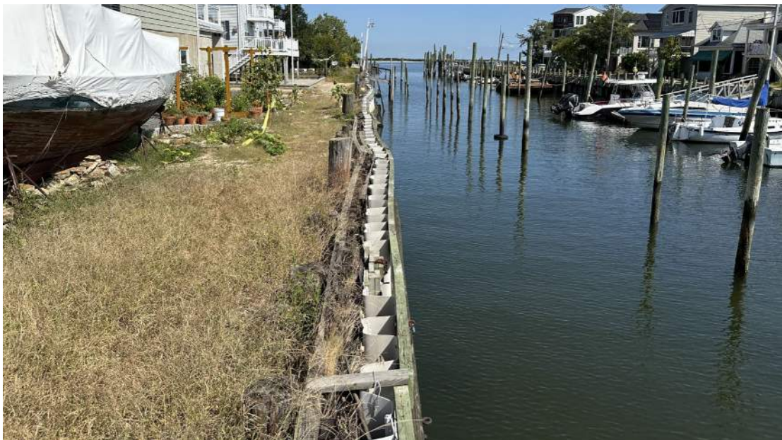
Photo 31: Section C , Westerly Bulkhead, Bulkhead Line, View 1
