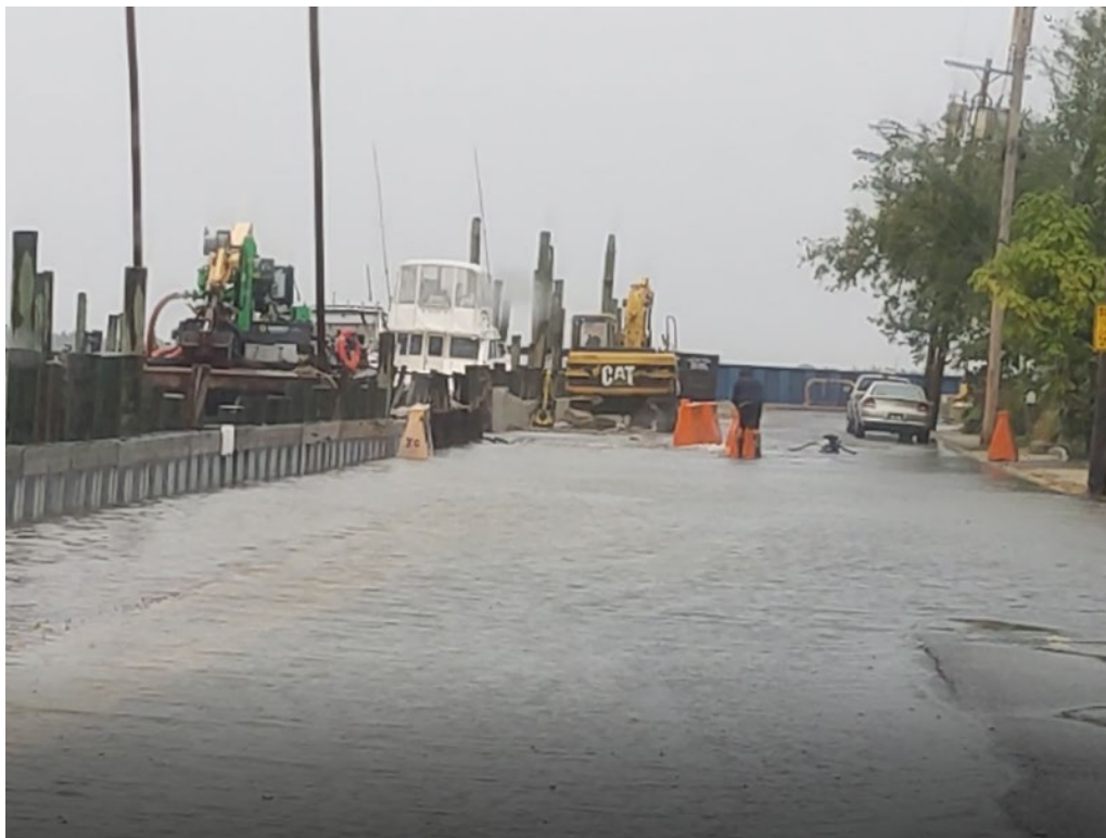
Flooding observed at Washington Avenue (10-3-2022)(Provided by William Brunt)
