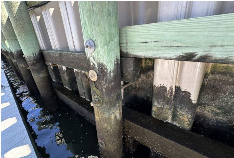
Photo 5: Section A , Easternly Bulkhead Water Lap Connection, View 1
