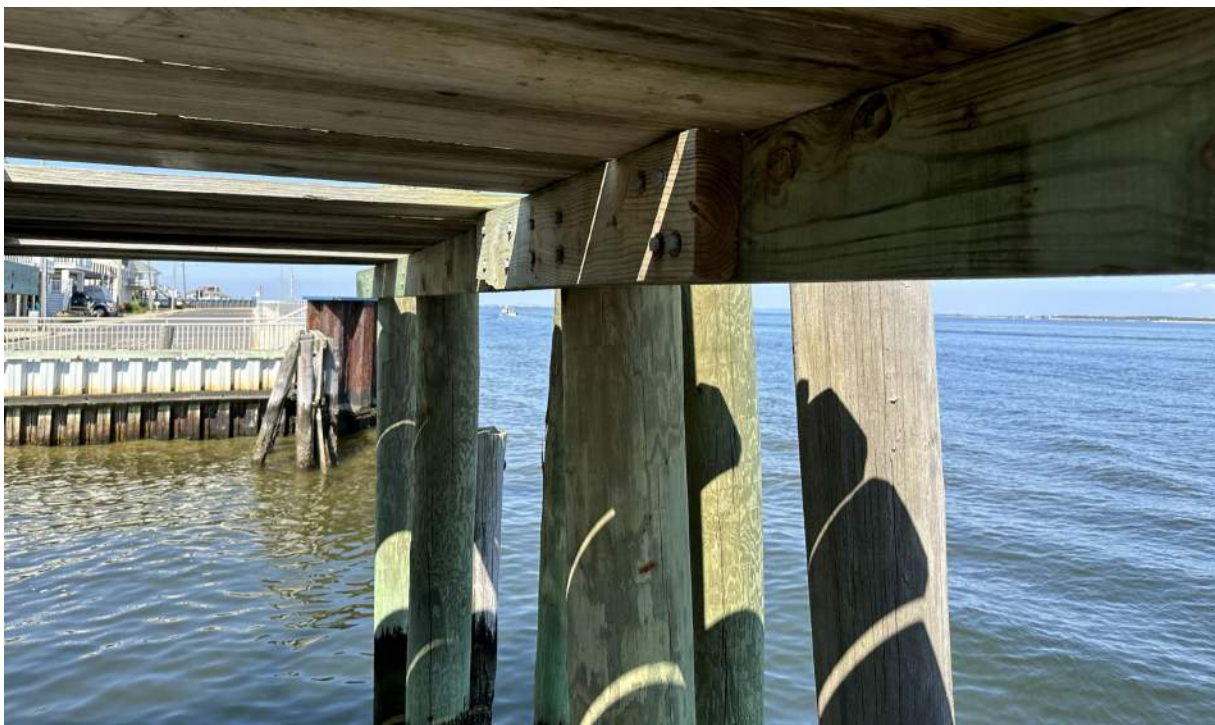
Photo 40: Section D , Easternly Dock, Girder to Pile Connection, View 1
