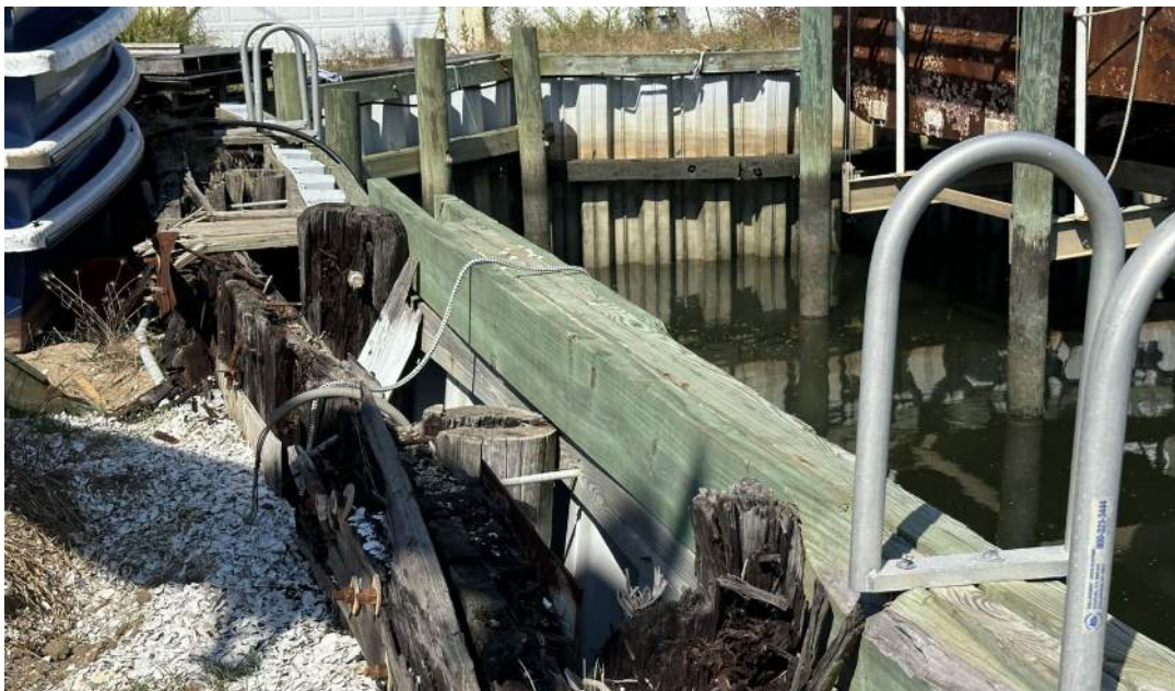
Photo 15: Section B , Southernly Bulkhead, Corner with Westerly Bulkhead, View 1
