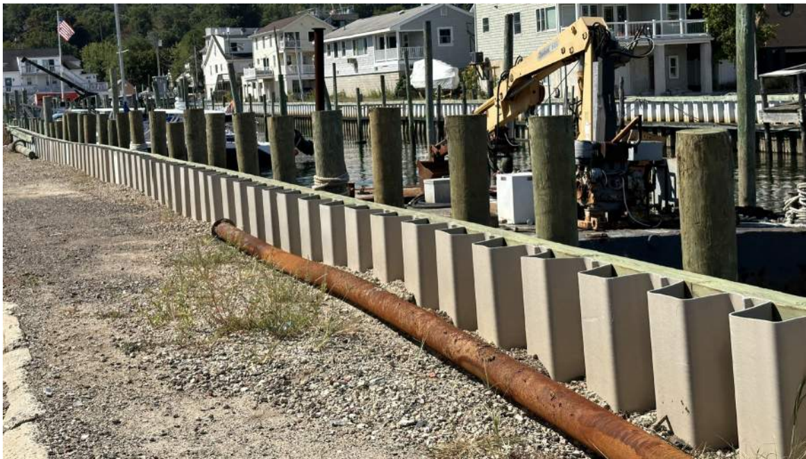
Photo 7: Section A , Easternly Bulkhead, View 1
