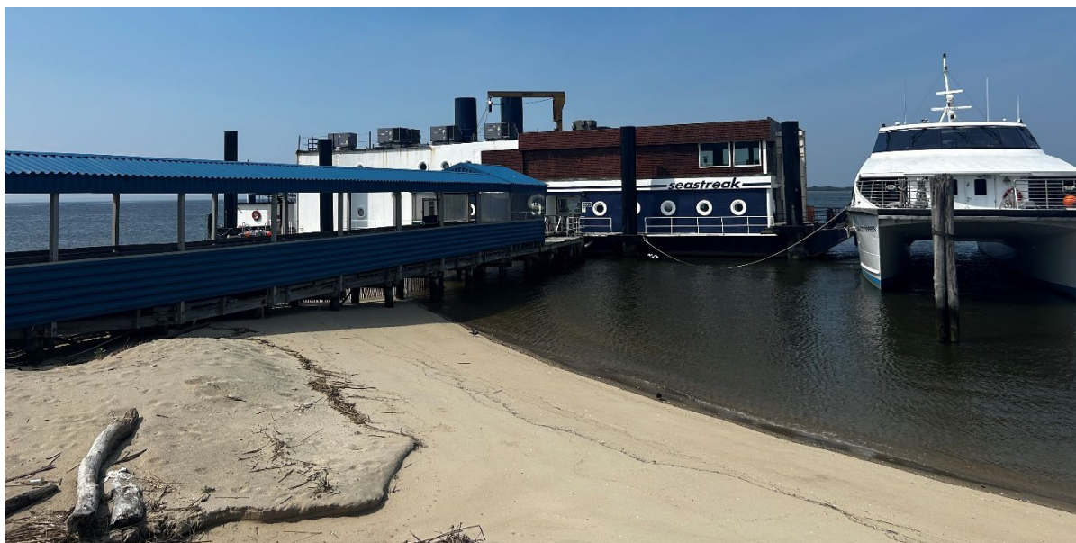
Seastreak ferry terminal.
