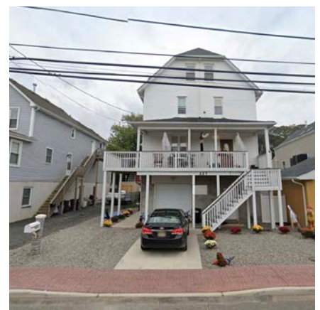
An example of a generous front porch on the Lowest Floor.
