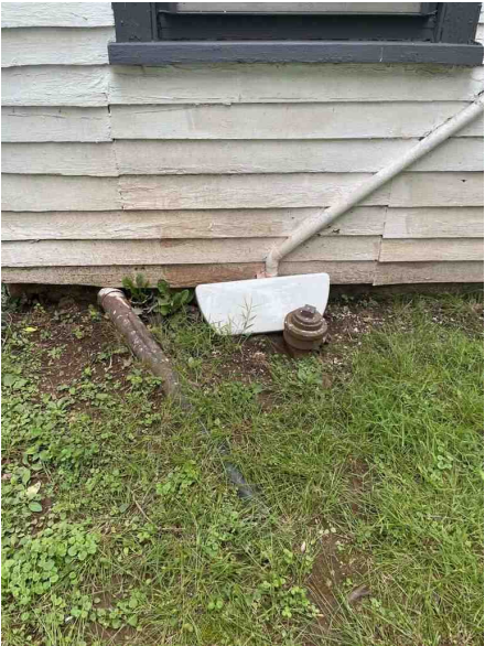
DEFERRED MAINTENANCE PVC PIPE PROTRUDING GROUND
