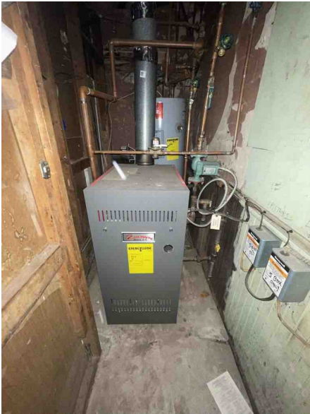
UTILITY CLOSET BOILER/WATER HEATER
