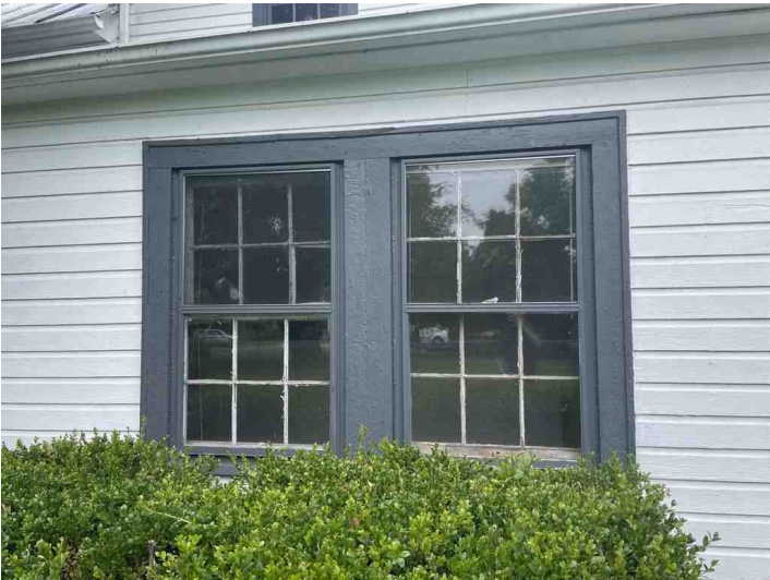
WOODEN SINGLE-HUNG WINDOWS WITH STORM SASH WOOD SIDING
