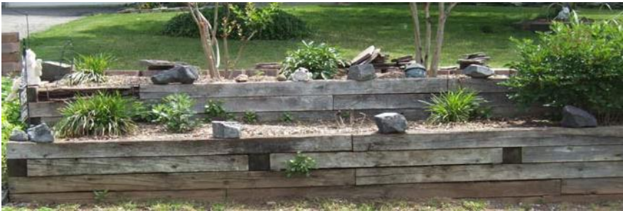
Wood Retaining Wall
