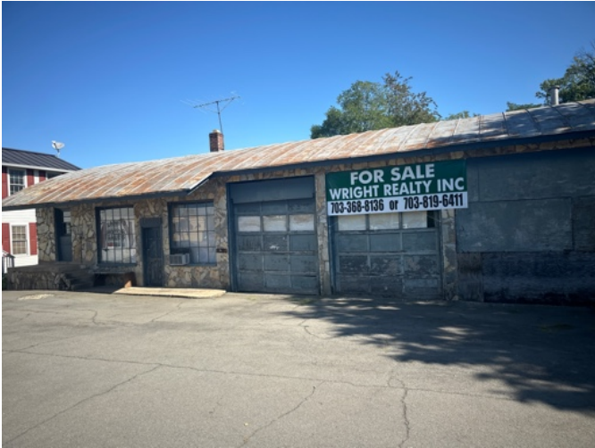
3.2) Walls, Ceilings, Floors
