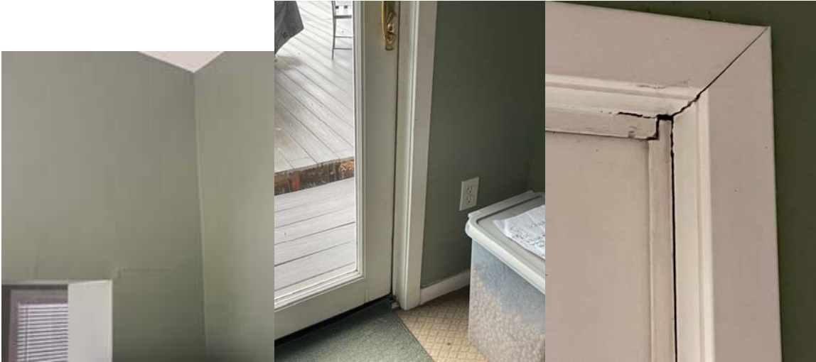
The sliding door and windows are not opening/closing properly anymore due to the shifting / bowing of the walls. These are some pictures of visual settling cracks and decay inside.
