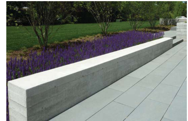
Commercial and Mixed Use Wall
