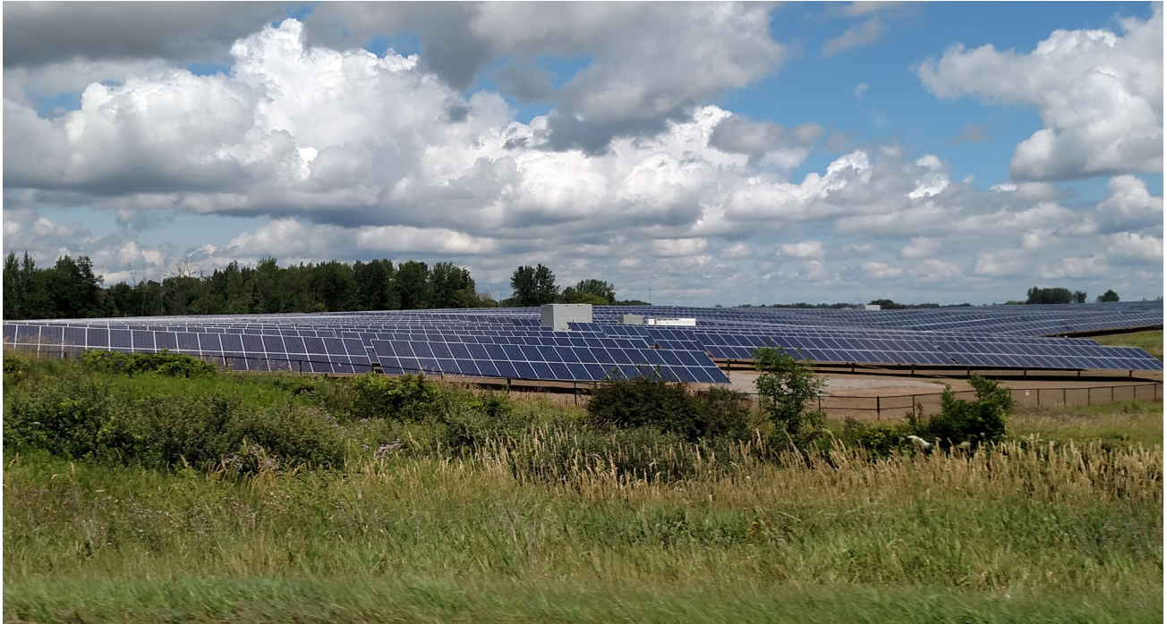
Lapeer Solar Park. Photo by Bradley Neumann.
