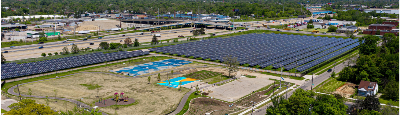
O'Shea Solar Park, Detroit. Photo by DTE Energy.
