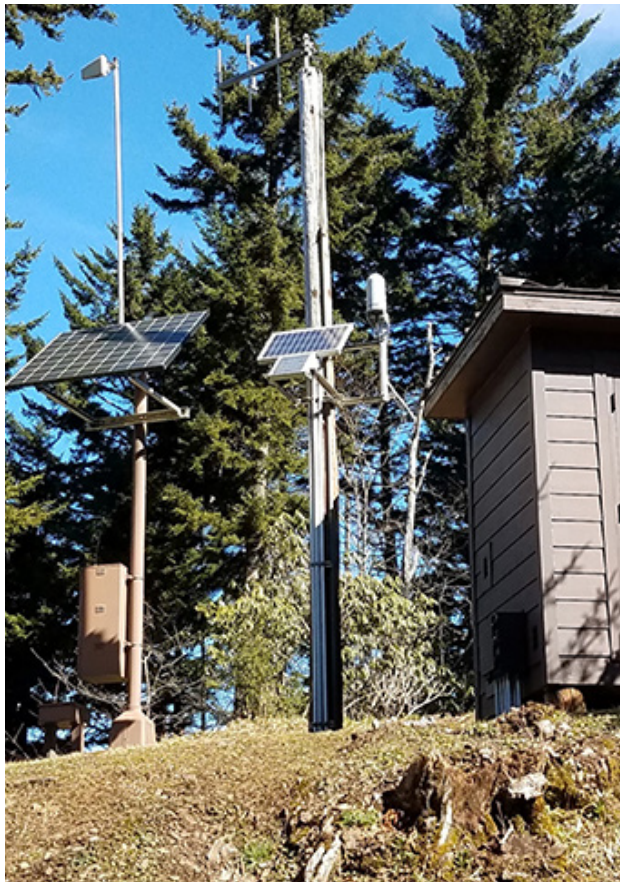
Accessory ground-mounted SES powering remote meteorological and communications equipment. Photo by Bradley Neumann.
