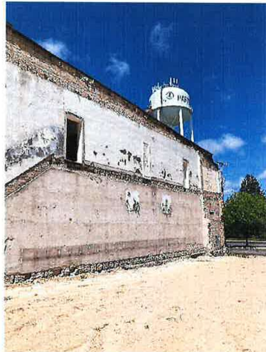
Photograph #8: Exposed Brick Shared Wall
