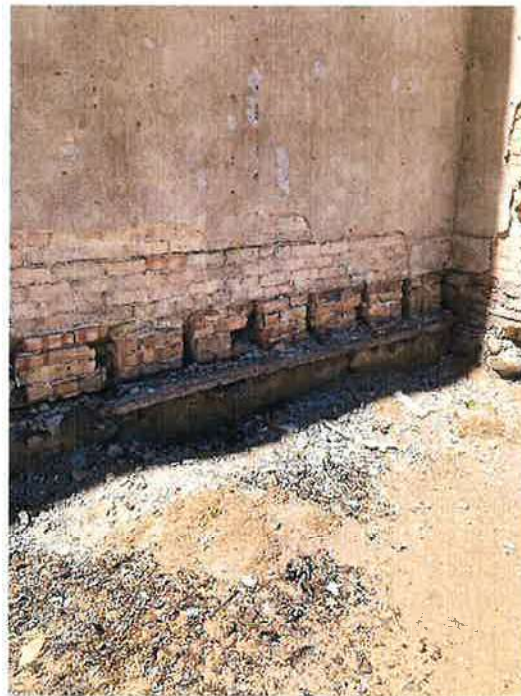
Photograph #11: Rotted Wood Plate
