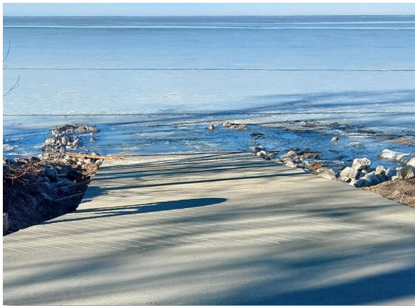
Fig. 16: Faro Springs Emergency Access
