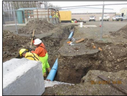
City crews repairing sanitary sewer system
