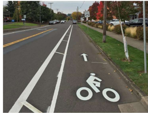
Photograph 4. Buffered Bike Lane
