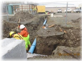
City crew repairing sewer system
