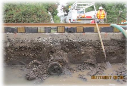
4th Street Railroad Project
