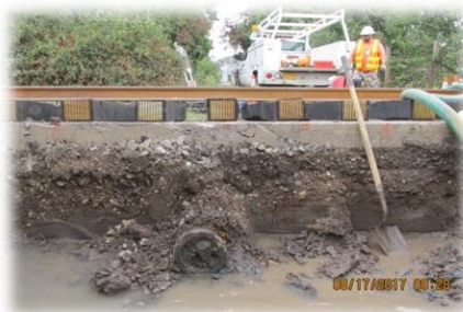
4th Street Railroad Project
