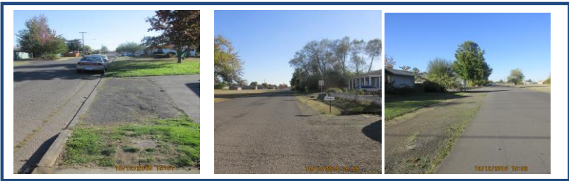
9th St. @ Burton, and nearby- 9 th & Territorial St. - SRTS Project
