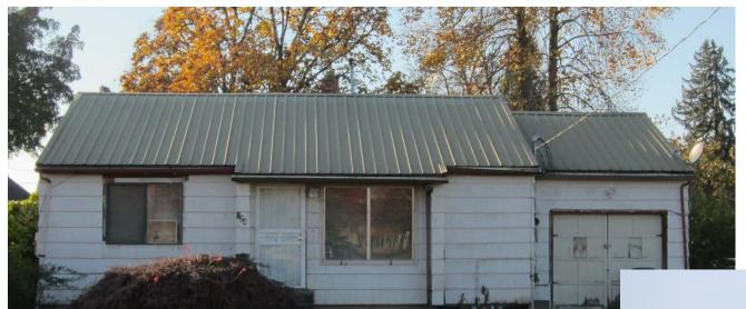
Original windows, siding in poor condition with lead based paint. We replaced with windows, siding, exterior doors and the project will continue with funds from the USDA program.
