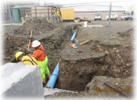
City crew repairing sewer system
