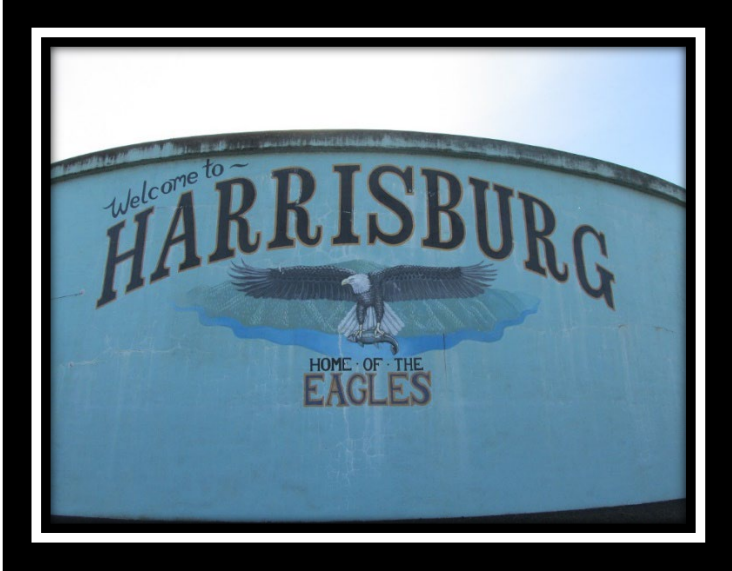
2 M Gallon Water Tank
