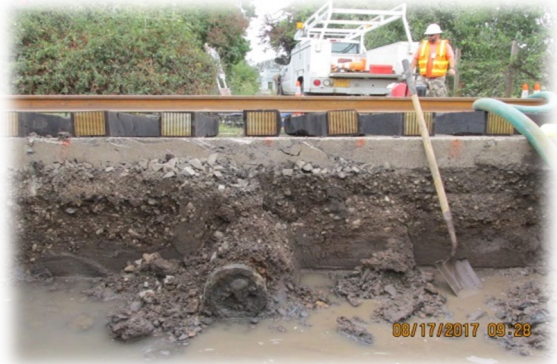
4th Street Railroad Project
