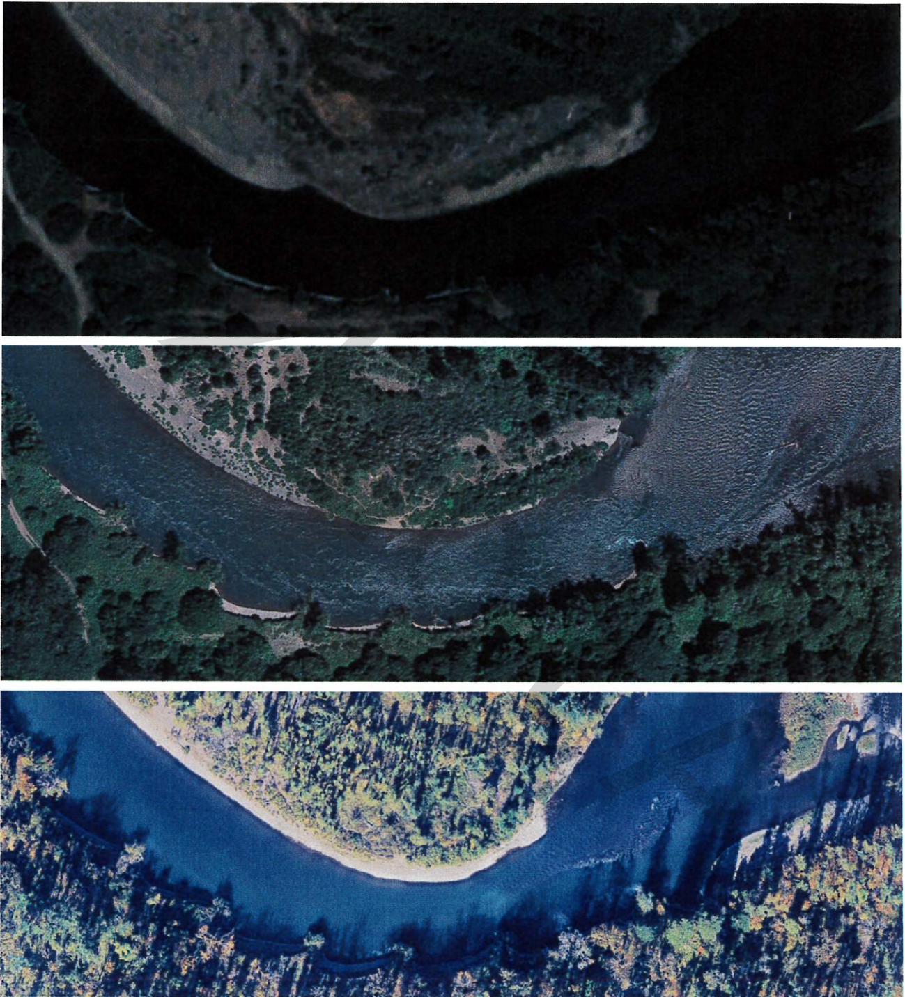
Figure 8: Aerial photographs (top – 2003, middle – 2014, and bottom – 2024) showing rock bendway weirs along the left bank outside bend (flow proceeding from right to left) constructed in the Middle Fork Willamette River upstream of Clearwater Park in Springfield, Oregon, that have been stable and functional according to conversations with ODFW.
