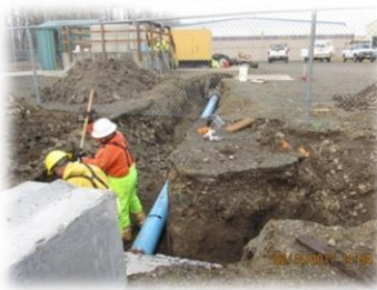
City crew repairing sewer system
