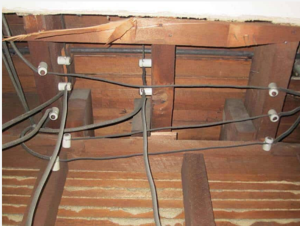
Knob and Tube wiring
