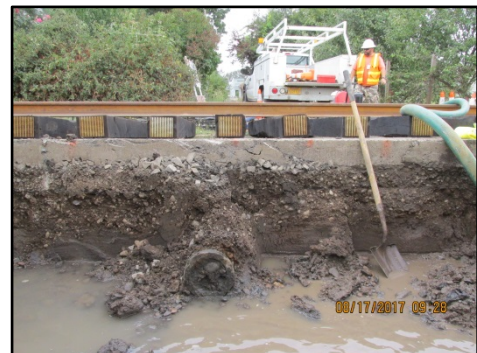
4th Street Railroad Project
