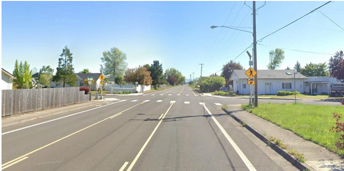
Photograph 2-2. Existing Enhanced Crossing on Diamond Hill Drive at 9 th Street
