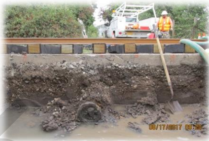
Figure 1 Water Line Replacement
