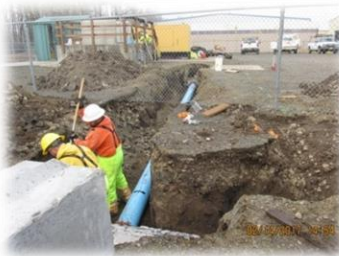
City crew repairing sewer system
