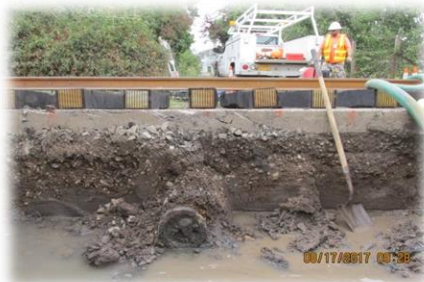
4th Street Railroad Project
