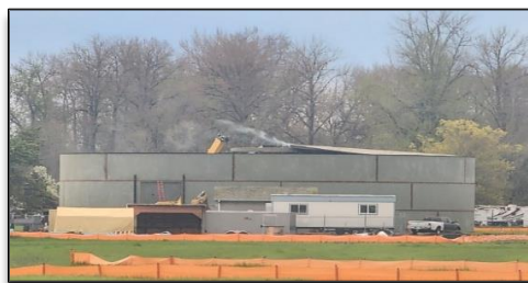
North Water Reservoir Under Construction 1
