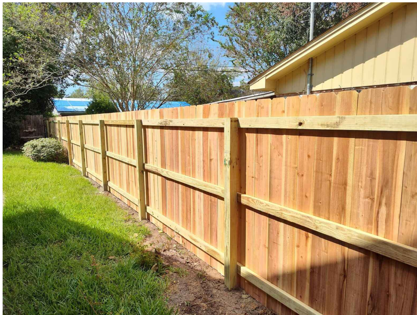
Size: 6' High, 8' Long Panels with Structural Members Facing Project Site
