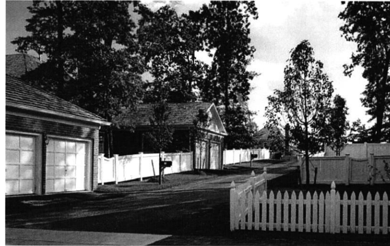
Garages with access from an alley
