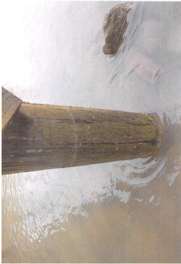
Bridge No. 0445 Br. Name Good River Date 05/17/19 Inspector McRae / Murray Frame 22 P3 DS pile vertical splits File P5170625.JPG
