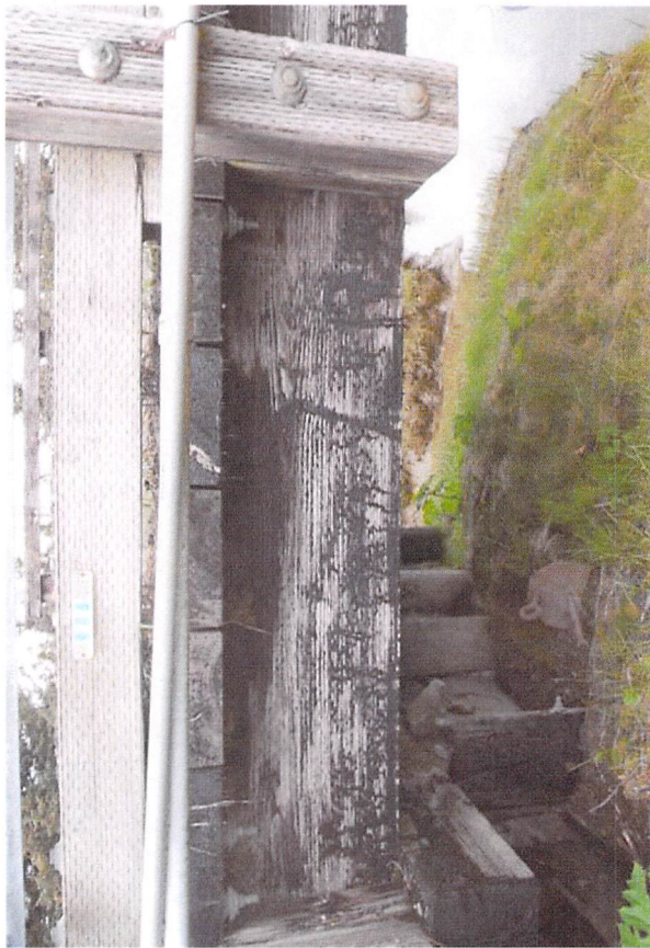
Bridge No. 0445 Br. Name Good River Date 05/17/19 Inspector McRae / Murray Frame 21 FE DS split in beam File P5170624.JPG
