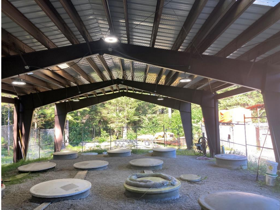
Figure 6. Wastewater treatment facility at Bartlett Cove
