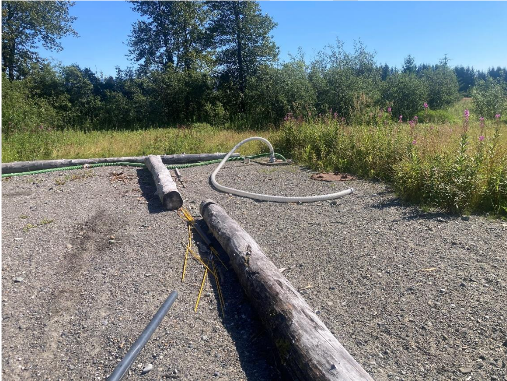
Figure 6. Caps of one of the septage holding tanks
