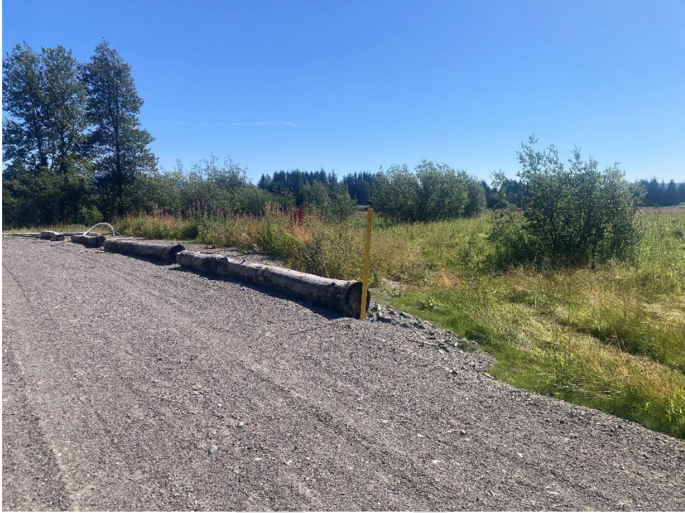
Figure 5. Location of the septage holding tanks
