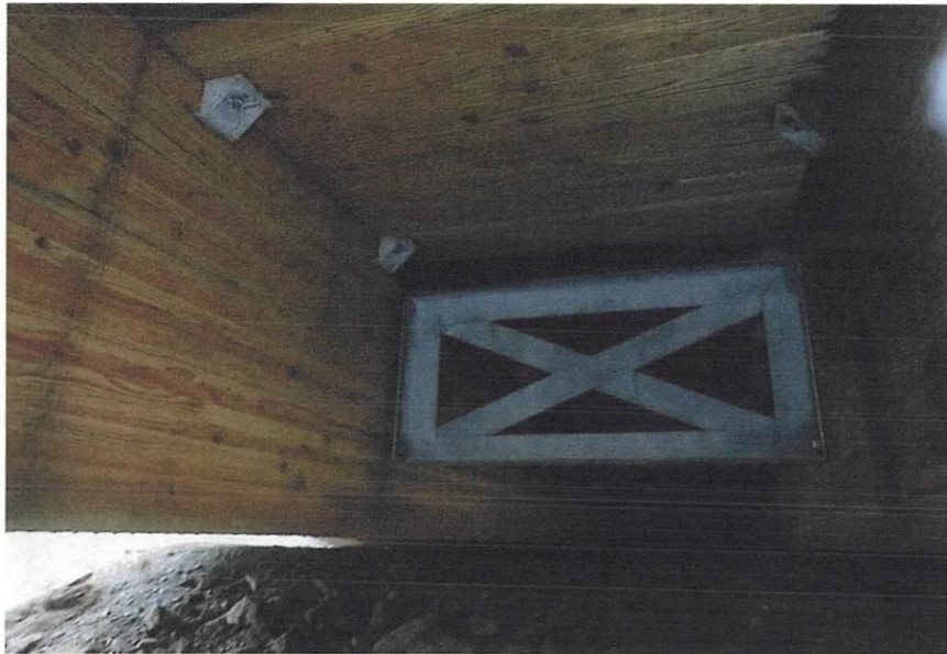
Bridge No. 2320 Br. Name Tong Road Bridge Date 05/19/21 Inspector Bailey / Daugherty Frame 21 Typ. Diaphragm File P5191021.jpg
