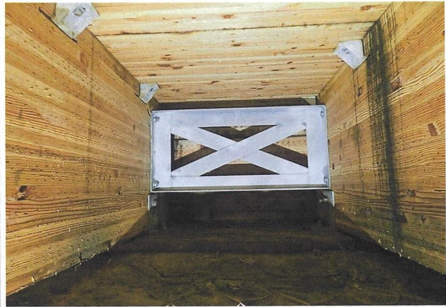
Bridge No. 2310 Br. Name Spruce Lane Bridge Date 05/19/21 Inspector Bailey / Daugherty Frame 18 Typ. End Diaphragm File P5191044.jpg
