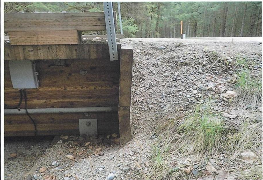
Bridge No. 2320 Br. Name Tong Road Bridge Date 05/19/21 Inspector Bailey / Daugherty Frame 18 NE DS Backwall Rotation File P5191029.jpg
