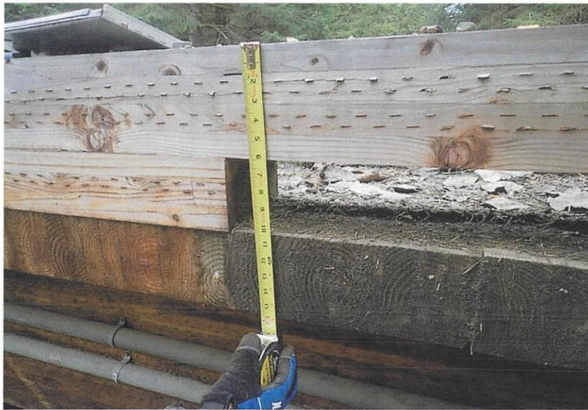
Bridge No. 2310 Br. Name Spruce Lane Bridge Date 05/19/21 Inspector Bailey / Daugherty Frame 13 Bullrail and Deck Thickness File P5191049.jpg
