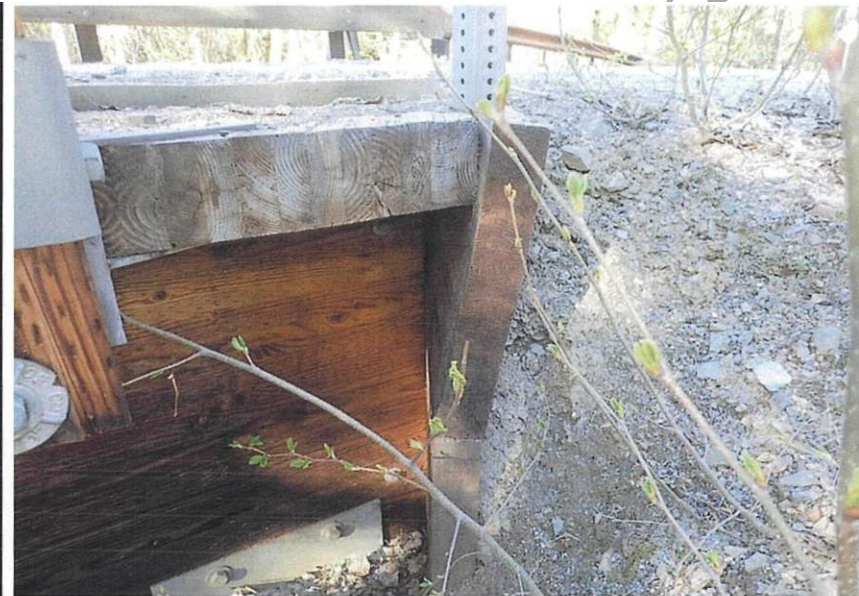
Bridge No. 2321 Br. Name Harry Hall Creek Bridge Date 05/18/21 Inspector Bailey / Daugherty Frame 22 NE DS Backwall Rotation File P5180997.jpg
