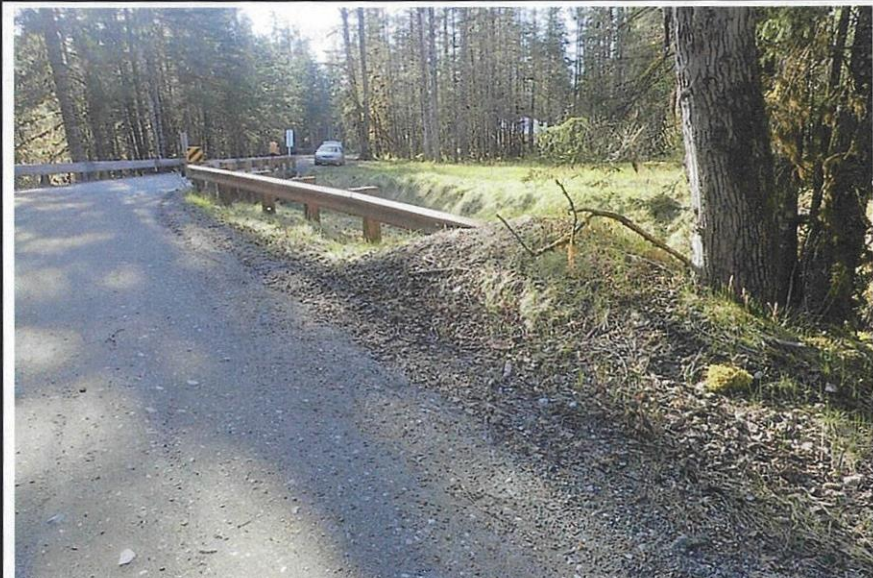
Bridge No. 2321 Br. Name Harry Hall Creek Bridge Date 05/18/21 Inspector Bailey / I Frame 12 Buried NE US End Treatment File P5180987.jpg
