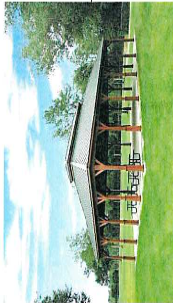
COMMERCIAL 20' X 40' HIP ROOF STYLE WOOD PAVILION KIT. AMERICAN LANDSCAPE STRUCTURES OR APPROVED EQUAL.
