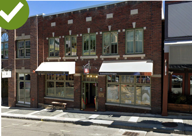
Windows occupy at least 50% of the first-story facade, and mullions are incorporated into window designs.
