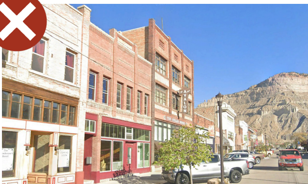
Three-story building without a third-story stepback.
