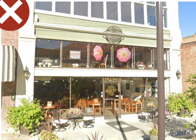
No defined material base at the bottom of the first-story windows. No incorporation of mullions.
