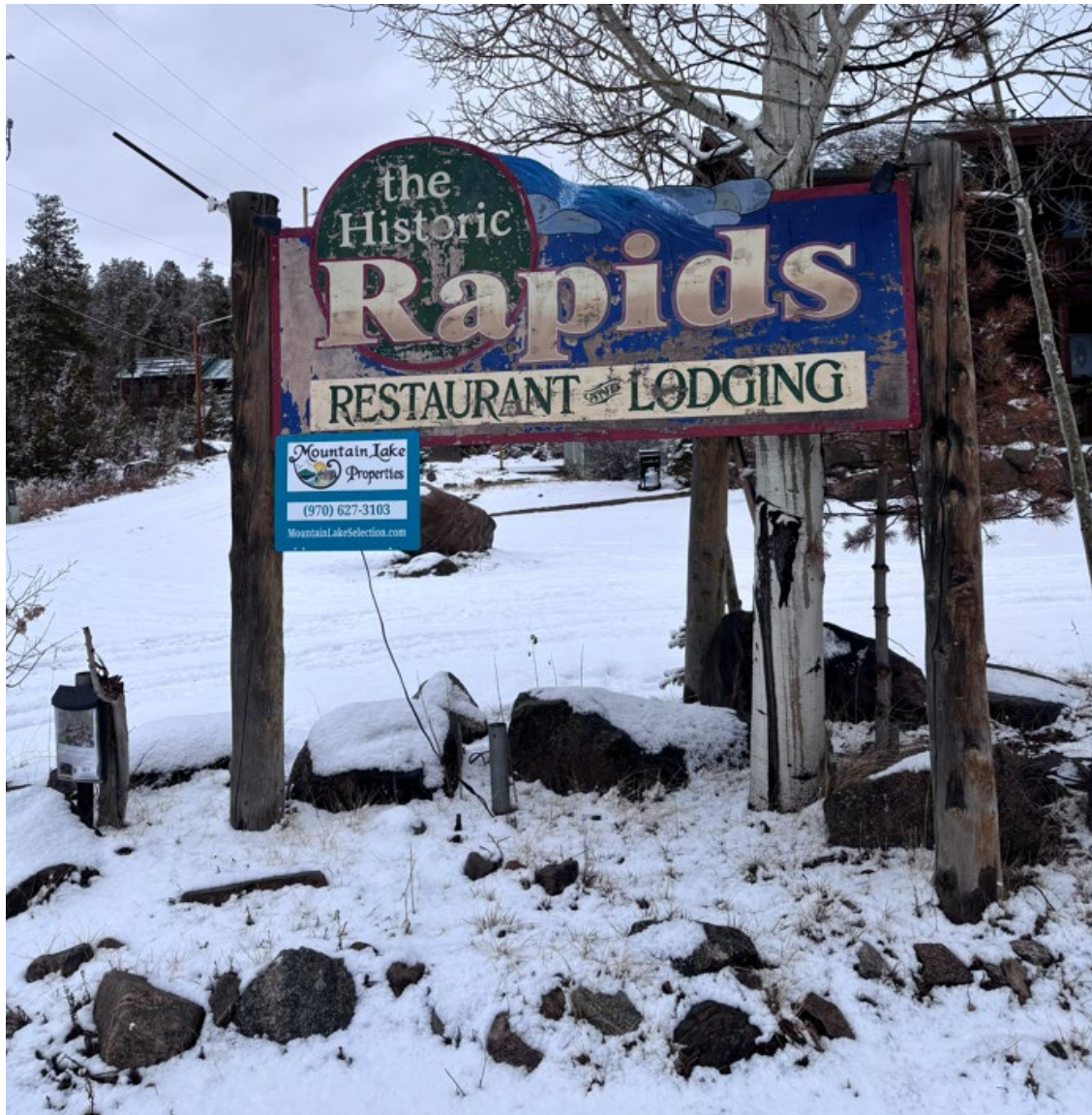
Southern facing sign on Martell property: 4' x 8' = 32 sq. ft. Needs attention: sign is faded/paint is peeling off, the right signpost is rotted and needs to be replaced.
