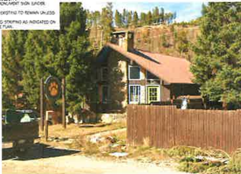
EXISTING BUILDING PHOTO
