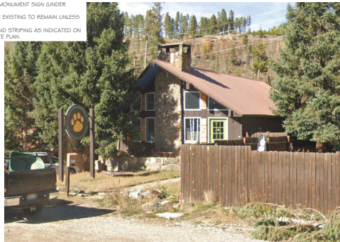
EXISTING BUILDING PHOTO
