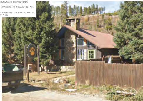
EXISTING BUILDING PHOTO
