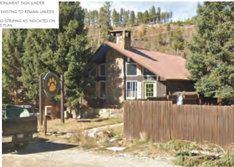
EXISTING BUILDING PHOTO
