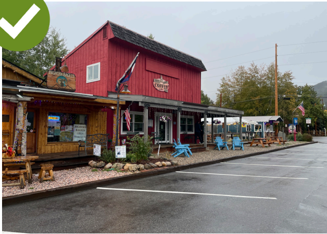
Parking spaces constructed within the ROW directly adjacent to the subject property.
