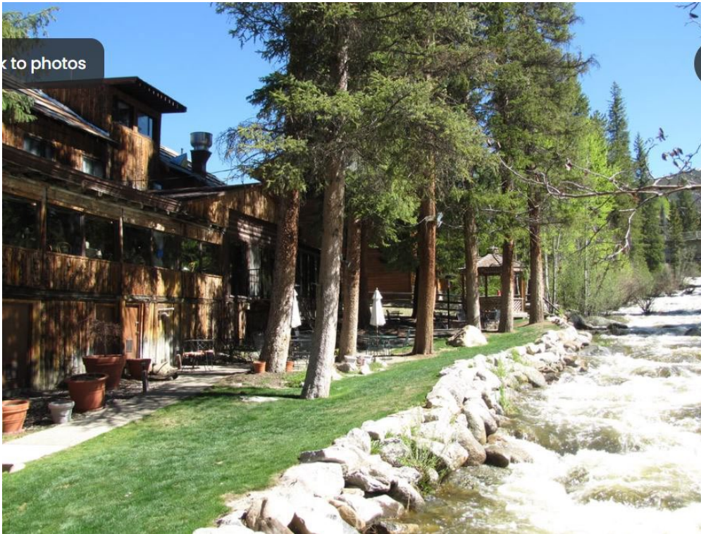
Figure 4-2014 thick lawn after the 2011 shoreline reinforcement
