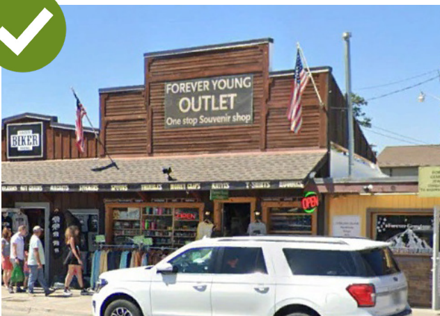
Flat roofs feature a false parapet.
