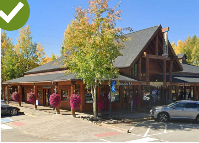
Development incorporates structured cover over the boardwalk.
