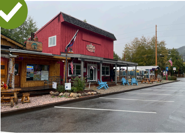
Parking spaces constructed within the ROW directly adjacent to the subject property.
