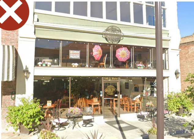
No defined material base at the bottom of the first-story windows.
