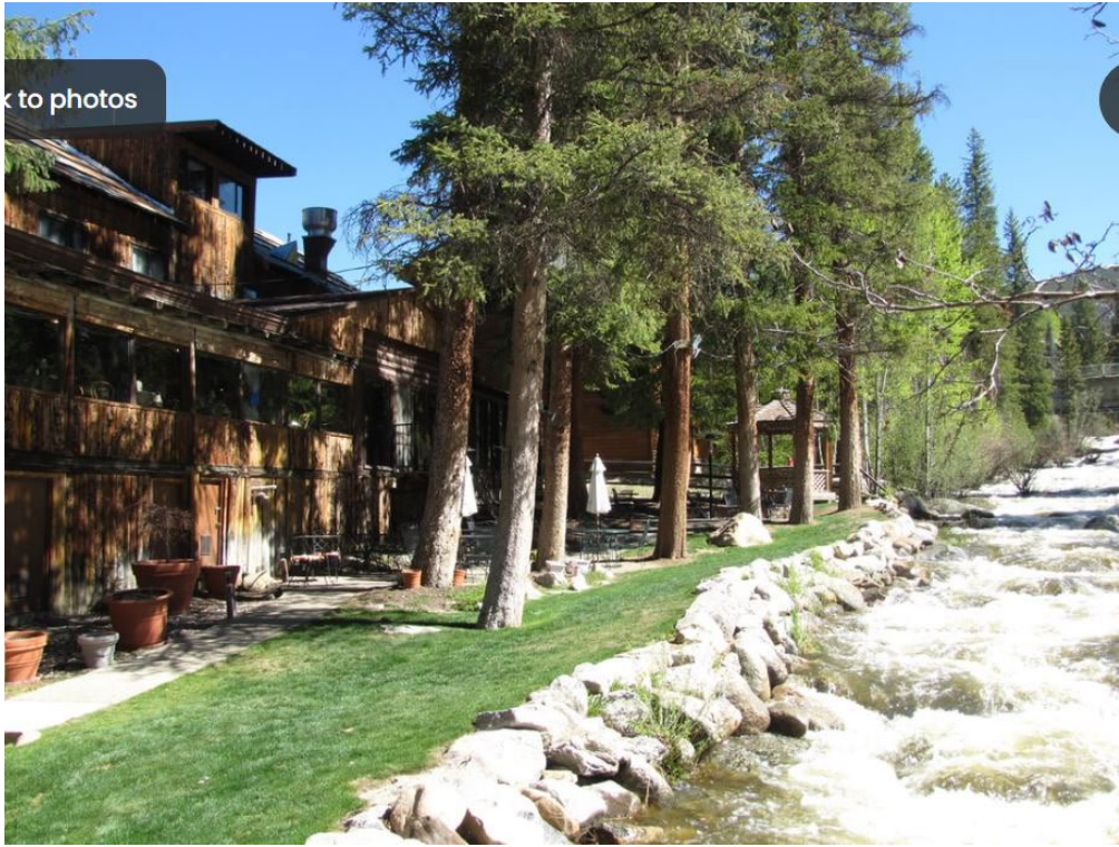
Figure 4-2014 thick lawn after the 2011 shoreline reinforcement
