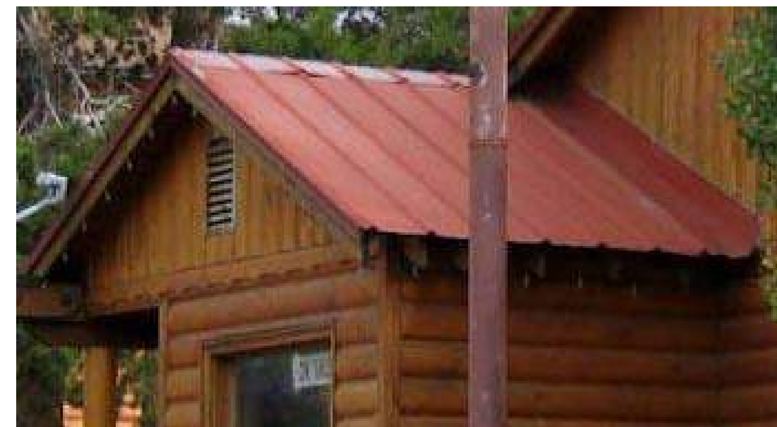
STANDING SEAM ROOF TO MATCH EXISTING
