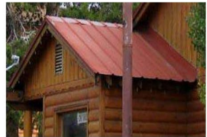
STANDING SEAM ROOF TO MATCH EXISTING
