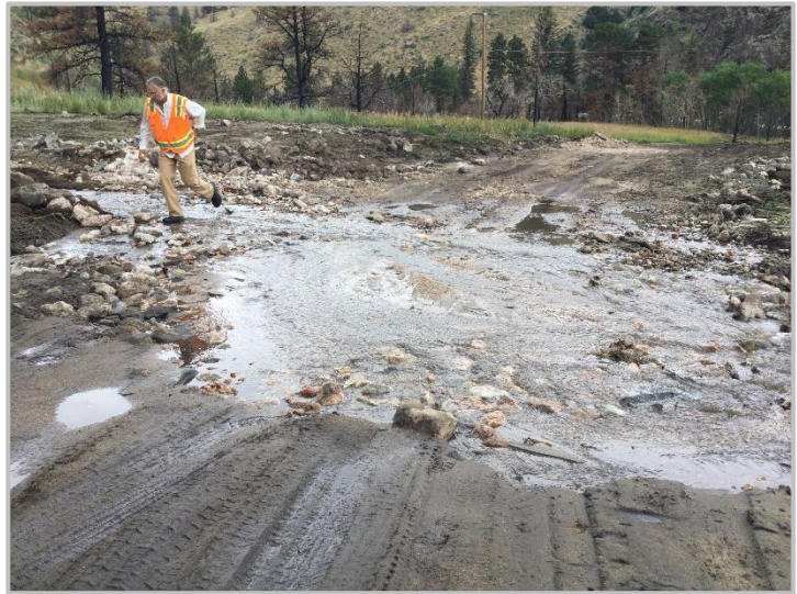
Figure 4: Road damage resulting from increased runoff generated in a post-fire watershed during a 2021 summer storm event.
