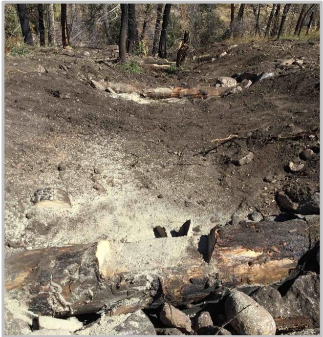
Figure 7: LWM Stabilization installation constructed in the Fall of 2021 in the CLP watershed.
