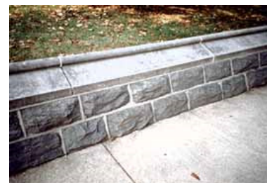
Caulking was inappropriately used here in place of mortar on the top of the wall. As a result, it has not been durable. Photo: NPS files.
