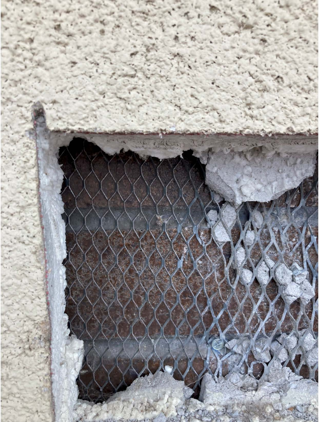
Test spot of uncovered brick
