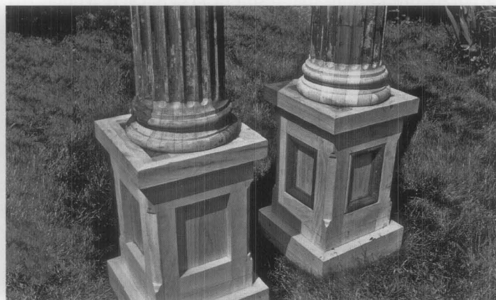
Figure 10. This nineteenth century porch column is made of wood staves, similar to the way a wood barrel is put together. After replacing the torus and making dutchman repairs to the apophyge along the base, the column and pedestal are ready to be reinstalled on the porch. Photos: NPS files.
