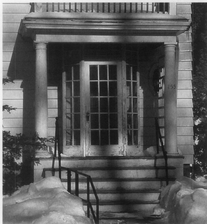
Figure 13. Particularly in New England, there is a cold weather tradition of installing temporary glass and wood panels at entrance doors, thereby creating an enclosed vestibule. These enclosures with their small divided lights were generally removed in the spring.
