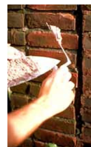
Soft mortar for repointing. Photo: John P. Speweik.
