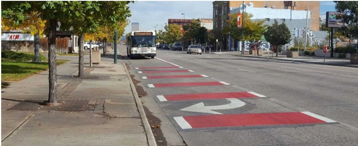
Figure 22: BAT Lanes (Source: Denver Streets Partnership)
